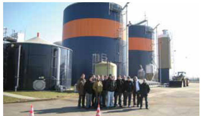
Biogasanlage in Rathenow
